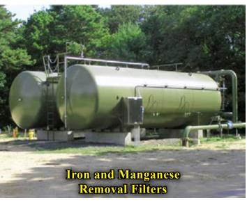
In areas where the groundwater naturally contains iron or manganese levels higher than the standard, sequestering agents such as polyphosphates may be added to control the iron and keep it in solution. We also use specialized iron and manganese removal filters, and employ strategies such as systematic flushing of water mains to reduce these naturally occurring metals. If any well exceeds the standard and does not have treatment, it is removed from service.
